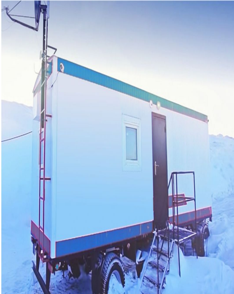
photo of the power station car-house
