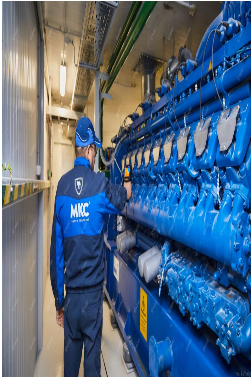
MWM gas piston plant. Photo by ISS Group of Companies
