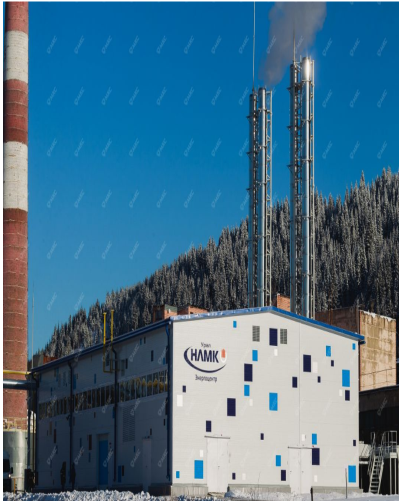
energy center produced by MKS Group for NLMK Revda plant
