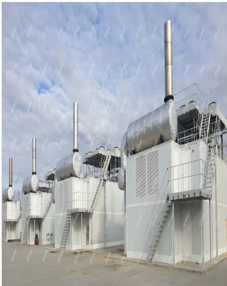
block modular design of gas piston power plant
