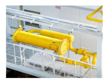
MKC Group of Companies has launched the production of gas purification plants called Cyclone. Innovative equipment will ensure gas pollutant extraction that enters the genset as efficiently and economically as possible, thereby increasing the service life of power plants. The fabrication of innovative products is deployed at MKC manufacturing area in Chelyabinsk. There can be produced Cyclone version with standard parameters, as well as customized version according to Customer's requirements.
