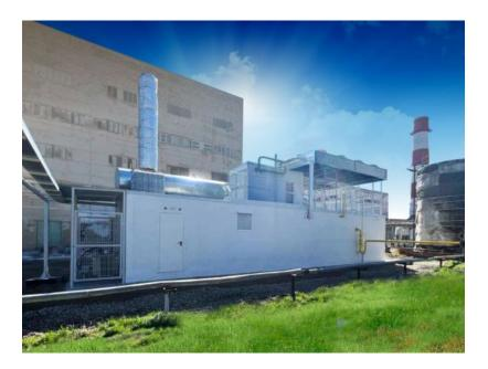
MKS Group commissioned a power center for the largest manufacturer in the Republic of Adygea. The 1.8 MW power plant will supply the oldest enterprise in the south of Russia with electricity and heat and will significantly increase the profitability of production.
