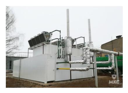
MKS Group completes construction of a block-modular power plant in the Yaroslavl region. The power center with a total capacity of 1200 kW will provide electricity and heat to one of the key enterprises of the Russian aviation industry. It is noteworthy that for the MKS Group this mini-HPP was the first facility to be implemented under an energy service contract.
