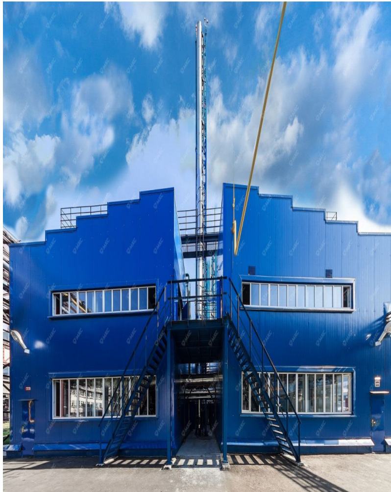
Trigeneration energy center of the chemical production plant Pigment JSC
