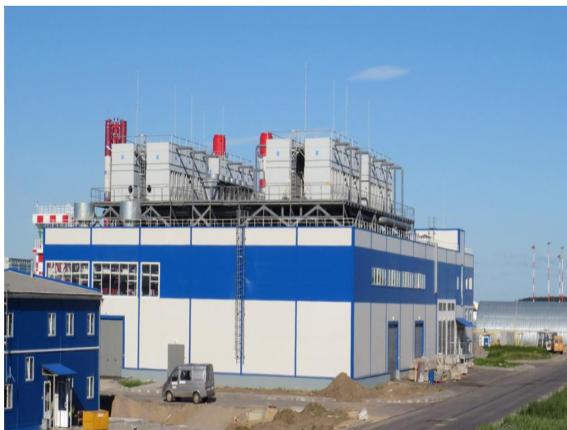
Pulkovo Airport Energy Center (St. Petersburg)
